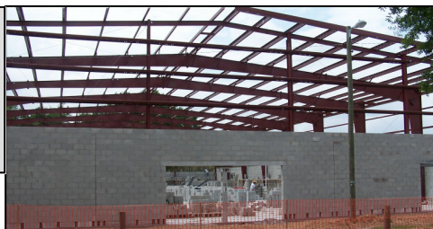
Our Gym Under Construction 2005
