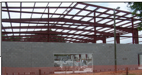
Our Gym Under Construction 2005
